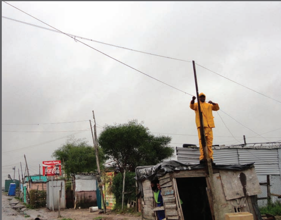
Houses built from scrap and illegal electricity connections, Sweet Home Farm
