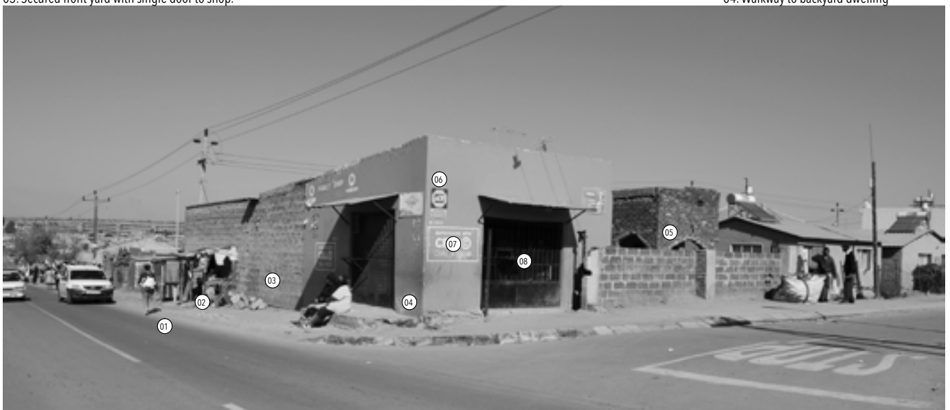
STREET ENTRANCE: A new boundary wall with gate secures the property from the street.
