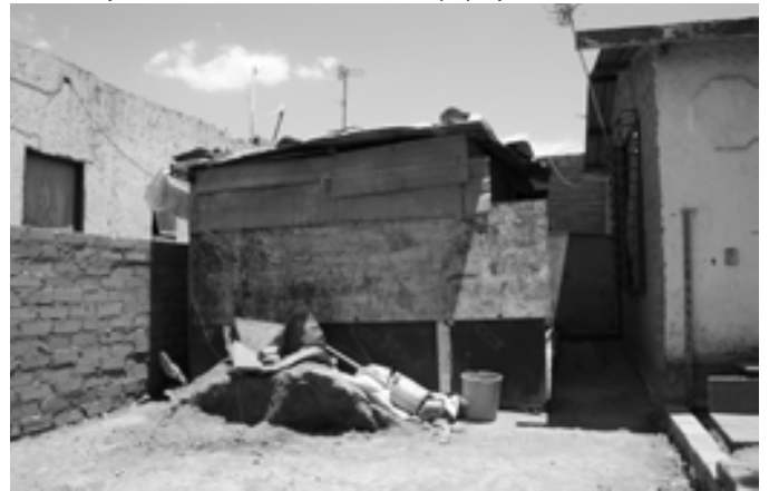
04. In-progress addition (furniture workshop for owner)
