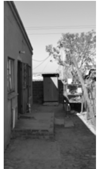
02. Outside (original) toilet
