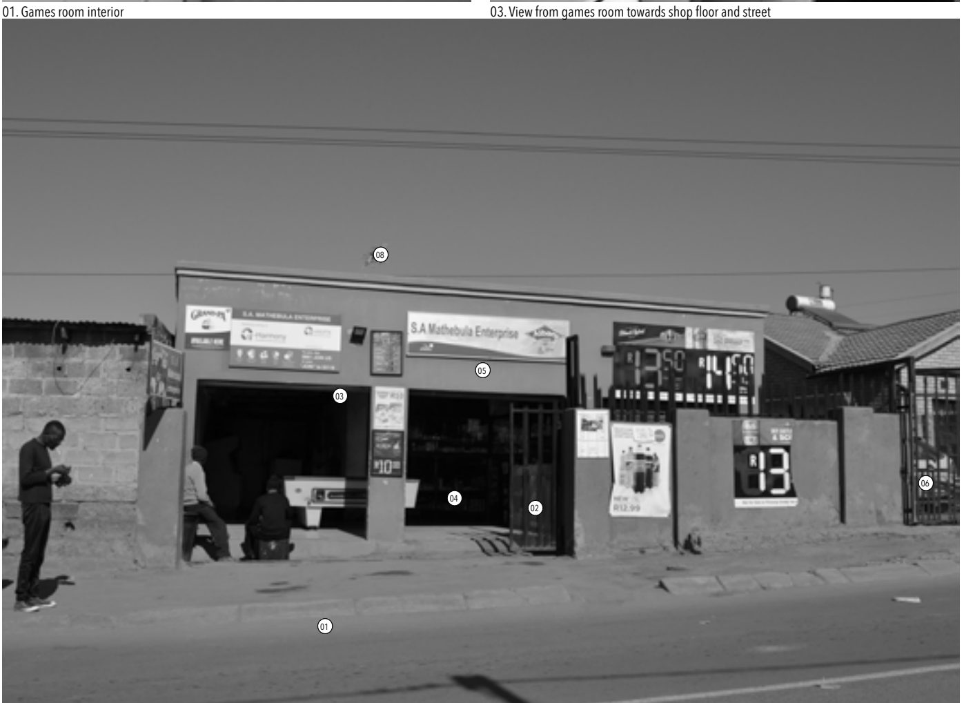
STREET RELATIONSHIP: Two large roller shutters and a sliding gate allow for the shop to have a good street relationship whilst maintaining security fixtures.
