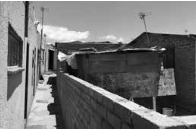
03. Passageway for circulation to individual residential units
